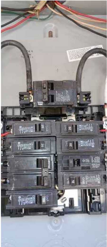
Branch Wiring Circuits, Breakers & Fuses: Branch Wire 15 and 20 AMP Copper
