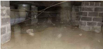
Floor Structure: Basement/Crawlspace Floor Dirt
