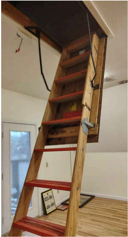
Attic Insulation: Attic Access Pull Down Stairs
