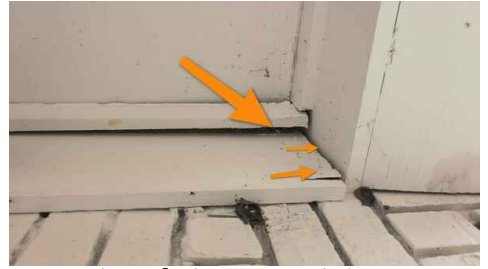
Separation of trim near attic in carport
