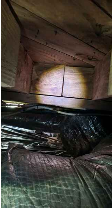
Floor Structure: Basement/Crawlspace Floor Dirt, Black Polyethylene Plastic
