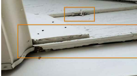
Some indications of wood deterioration on facia.
