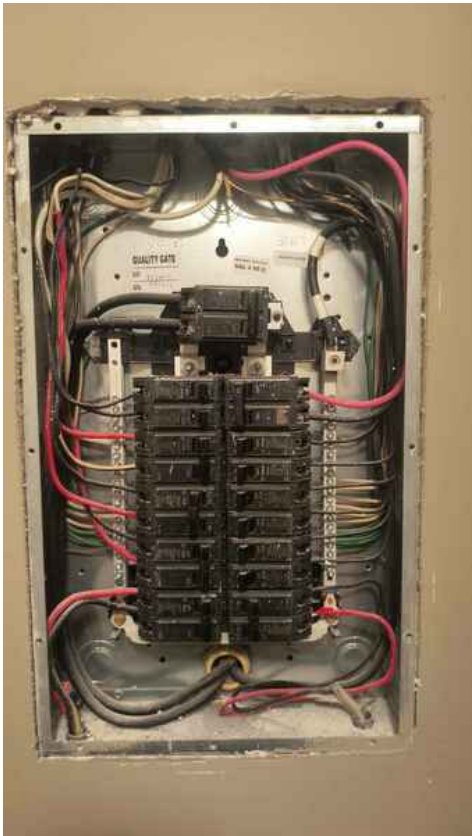
Branch Wiring Circuits, Breakers & Fuses: Wiring Method Romex
