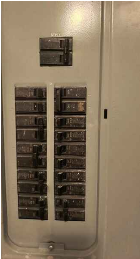
Branch Wiring Circuits, Breakers & Fuses: Branch Wire 15 and 20 AMP Copper
