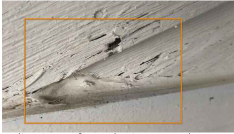
Indications of wood minor wood on Facia, in several areas.
